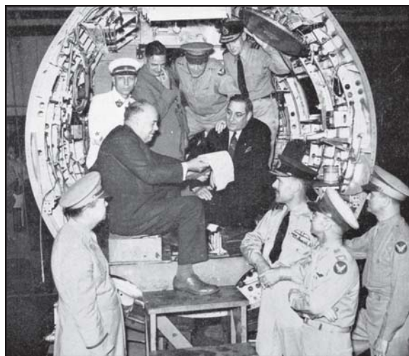
Three air force chiefs, Arnold of the USA, Belyaev of USSR and Evill of Great Britain, with Chrysler officials inspect B-26 construction progress.
